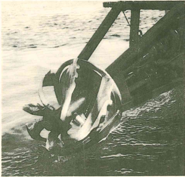
Working end of dredge
