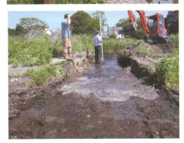
(Top) The WHAMM crew prepares to breach a berm of gravel and sand deposited by Hurricane Sandy, which prevented drainage. (Bottom) After the berm was breached, a channel was created to release the impounded waters that flooded the preserve and initiate normal tidal flushing.
